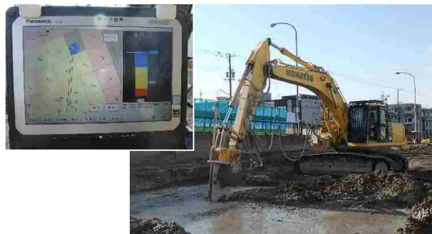
ICT地盤改良工
