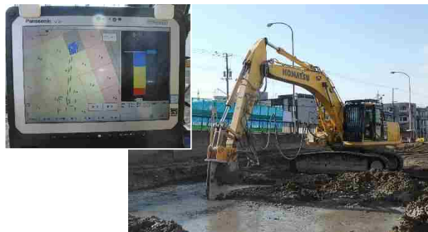
ICT地盤改良工
